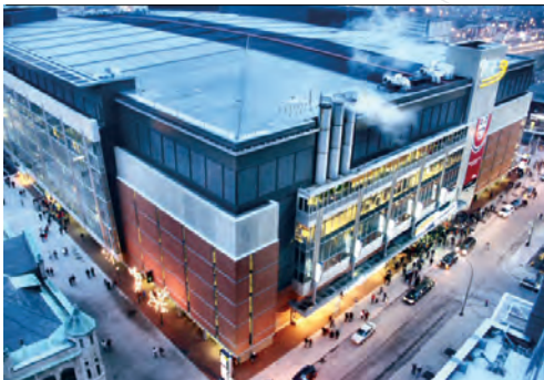
BELL CENTRE - MONTREAL, QUEBEC 251 CEILING HUNG POWDER COATED TOILET PARTITIONS 400 LOCKERS
